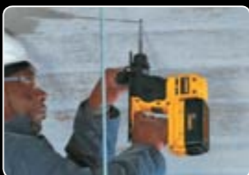
Drilling Anchor Holes in Ceiling For MEP Applications
